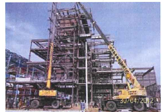
Erection Steam-Mud, Drum-Super Heater – Beame Boiler 782
