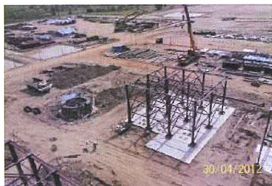
Erection Column ESP Gouting Boiler 783
