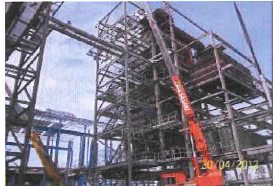
Erection Steam-Mud, Drum-Super Heater – Beame Boiler 782
